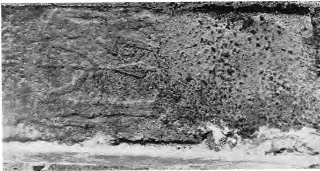
B. — View of pillar no. 8.
